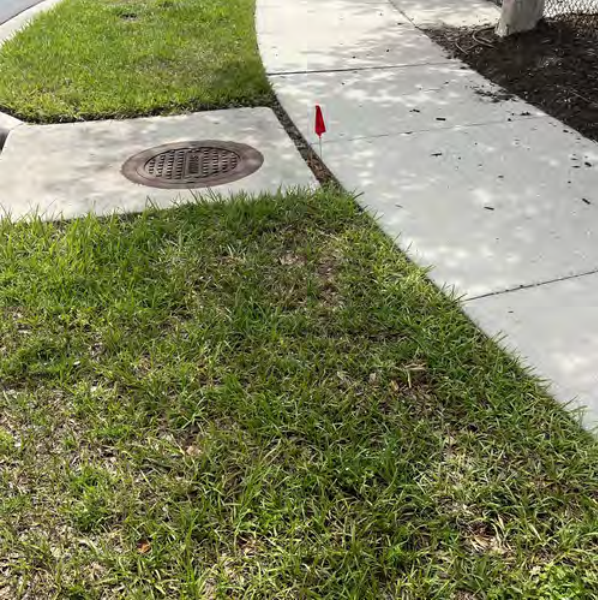
Zone #17 (Clogged Nozzle) - 06-08-26 10:21 am CDT
